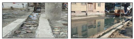
Photographs 4 and 5: Choked drains and overflowing drains in Narela IA, as observed during joint physical verification in January 2020
