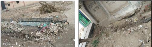
Photographs 6 and 7: Dumping of waste in drains and choked drains in Bawana IA, as observed during joint physical verification in December 2019
